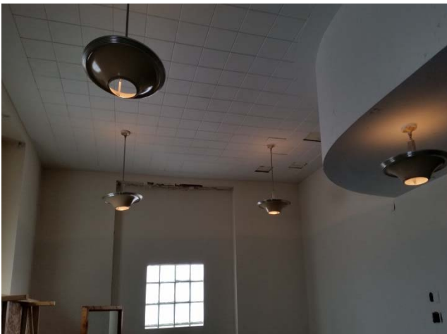
Light fixtures in a portion of the building
