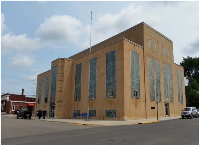
View of ECC facing NE from Harvey Street
